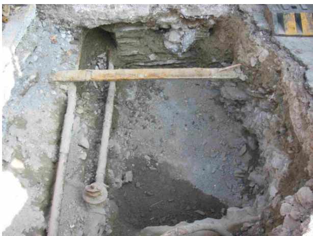
Links: Blick in die Startgrube.
